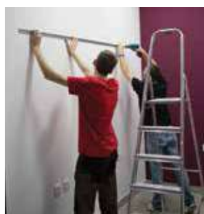
PHASE 1 Installation of the aluminium rail. Installation sur le rail en aluminium.
